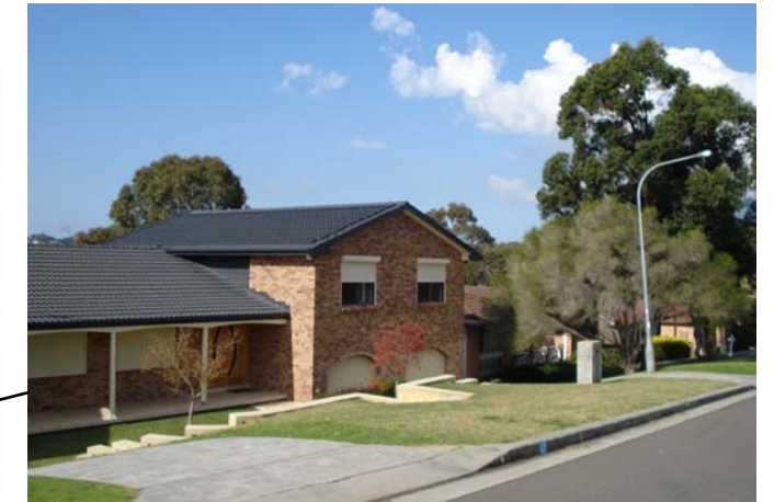
Typical built form in Penrose Subdivision fronting the site
