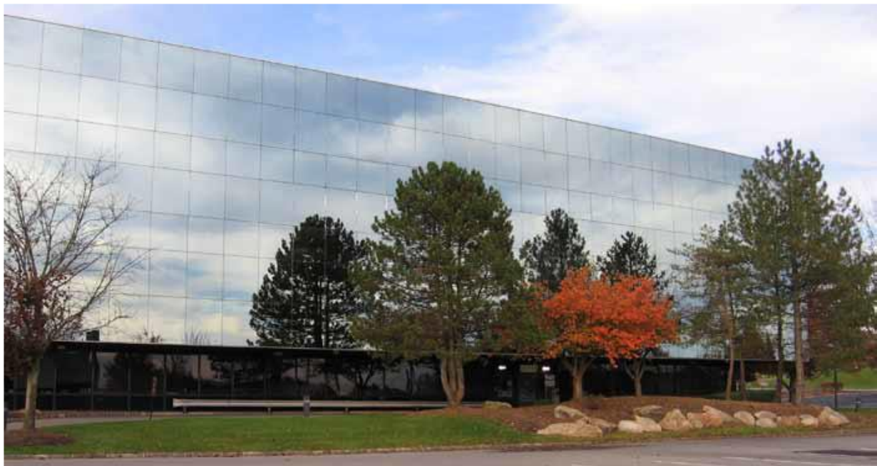
Figure 7: Example of a mirrored glass façade that can cause bird strike (from Sheppard 2011)
