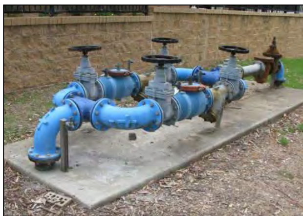
Figure 10 Balaclava Rd Main Meter
