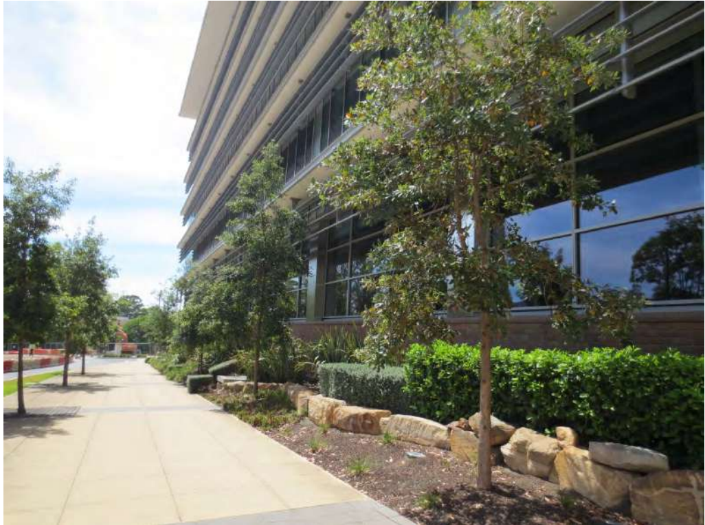
Figure 40 Cochlear Building frontage to University Avenue requires replacement planting.
