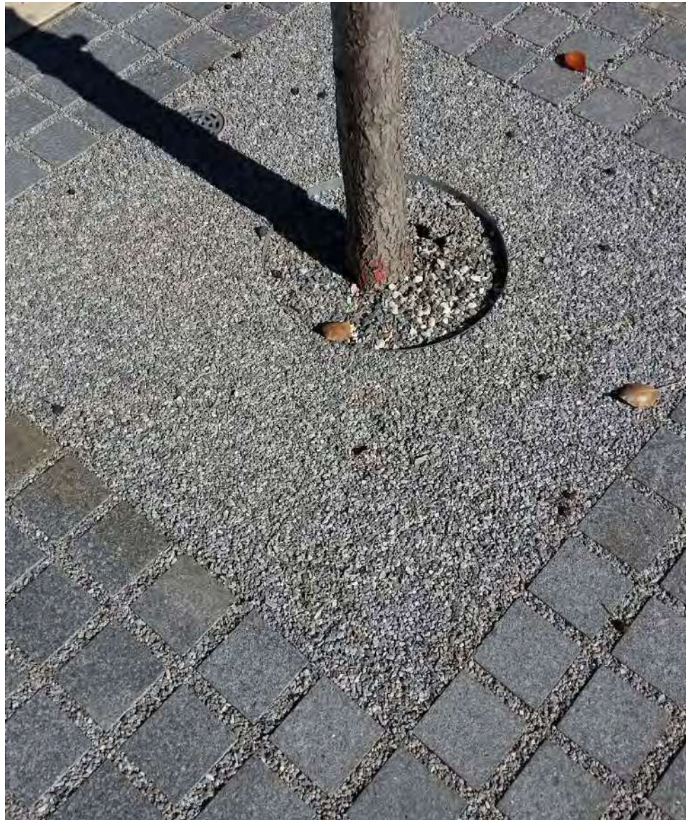
Figure 14 The metal surround should be removed well before the trunk outgrows the circumference.
