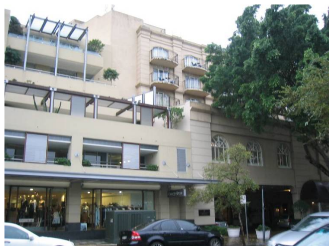
Figure 4. View looking north east to the Stamford Plaza Hotel The proposed design will link the hotel and mixed use developments to create a flowing retail experience with both internal and external retail shops.
