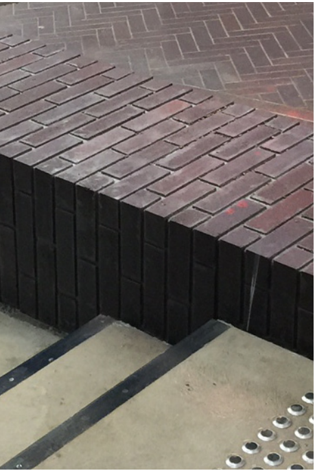
Brick wall - Kensington Street
