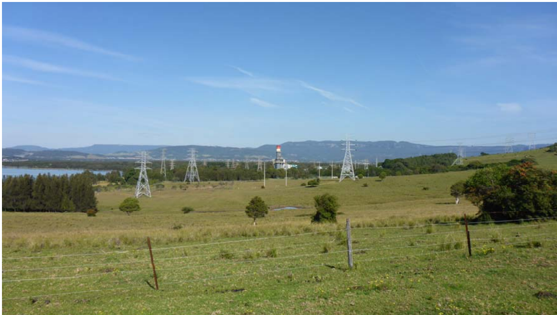
Photograph 35: a view toward the power station from the northern precinct
