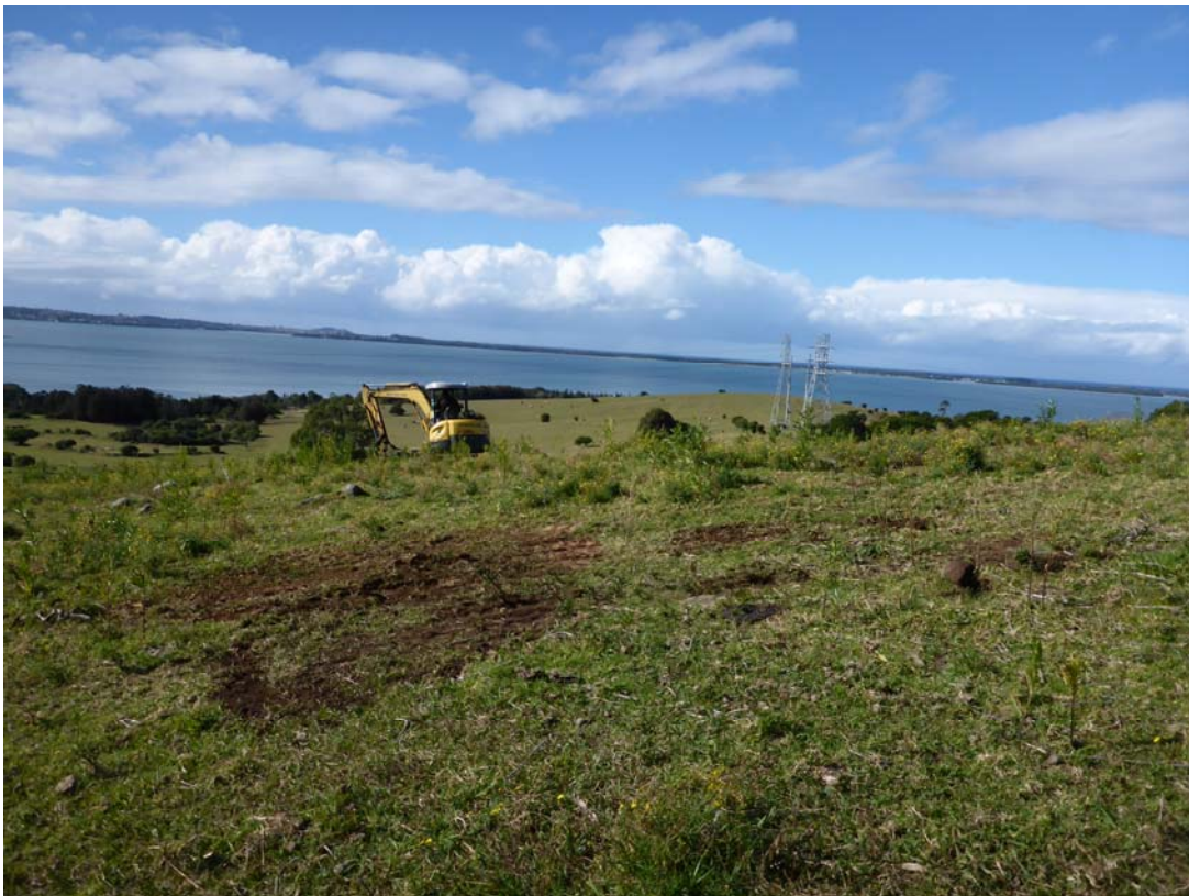
Photograph 30: View of backfilled test pit CTP106 (northern precinct).
