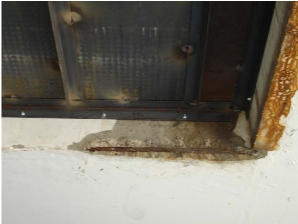
Photograph 23. Corroded Reinforcing Level 1 soffit
