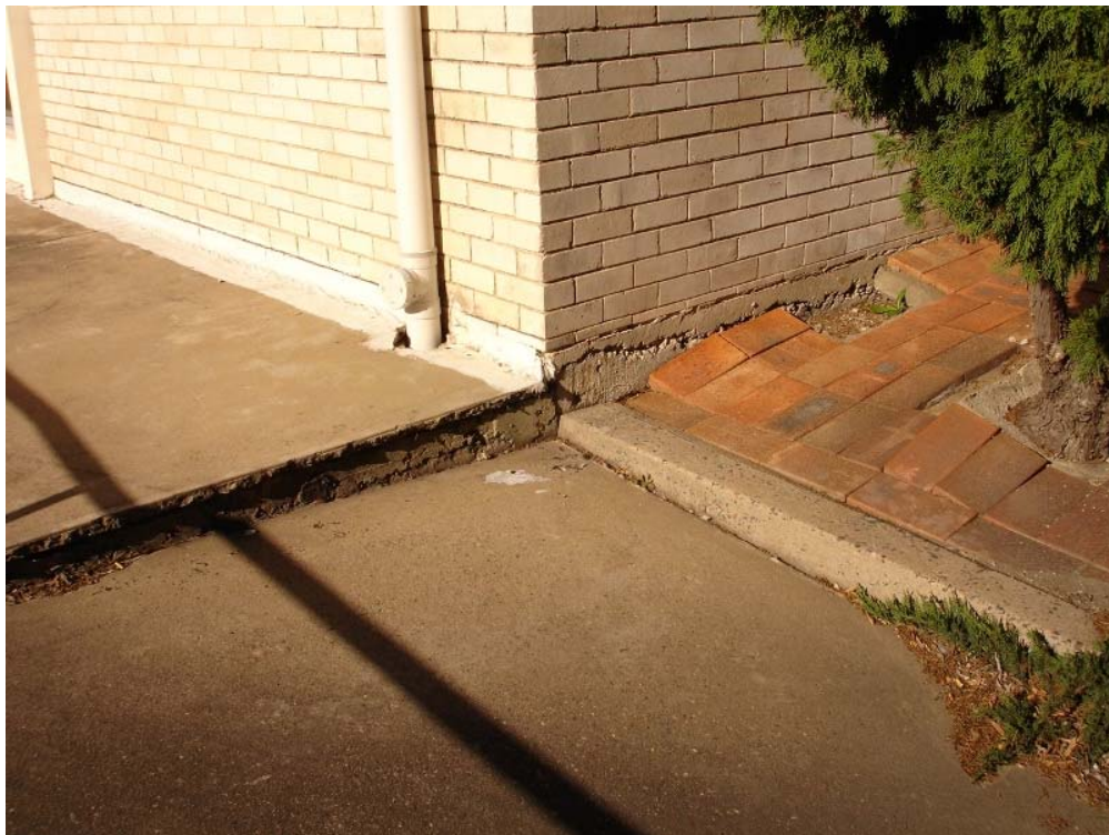
Photograph 14. Settlement of external pavement
