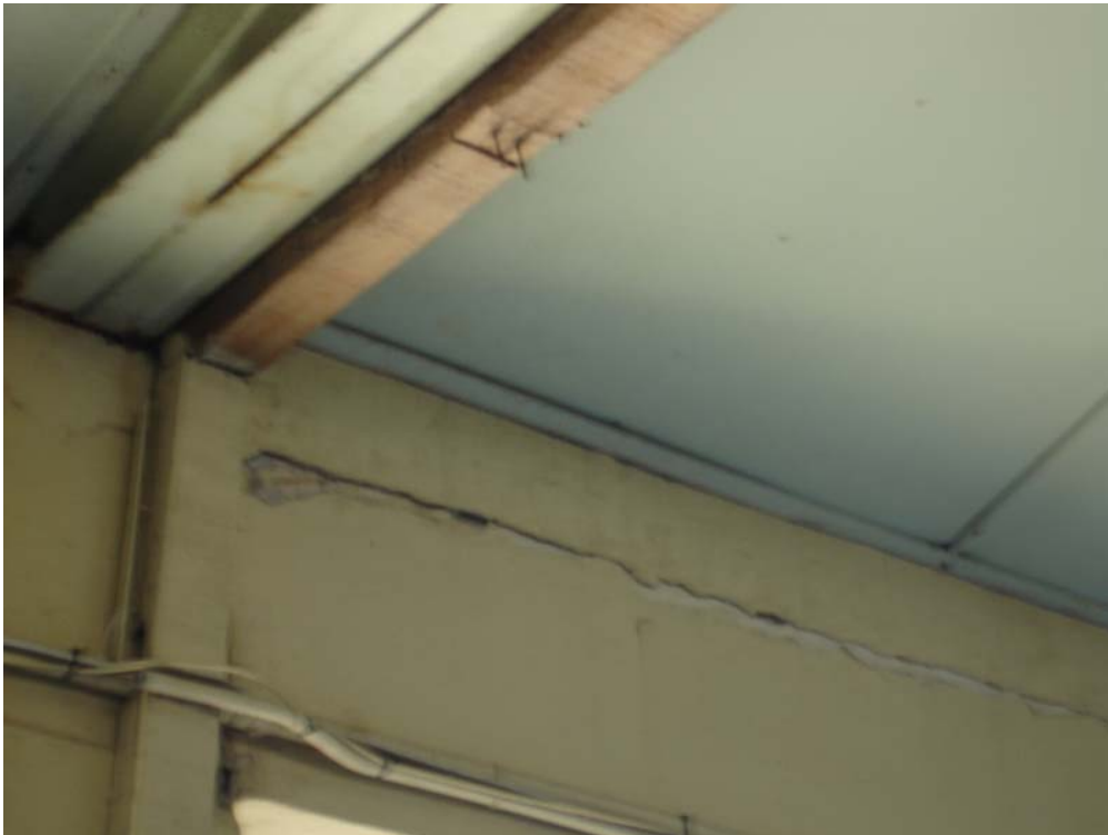
Photograph 43. Cracking masonry at roof level
