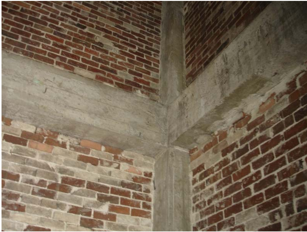
Photograph 49. Concrete and masonry framing to clock tower
