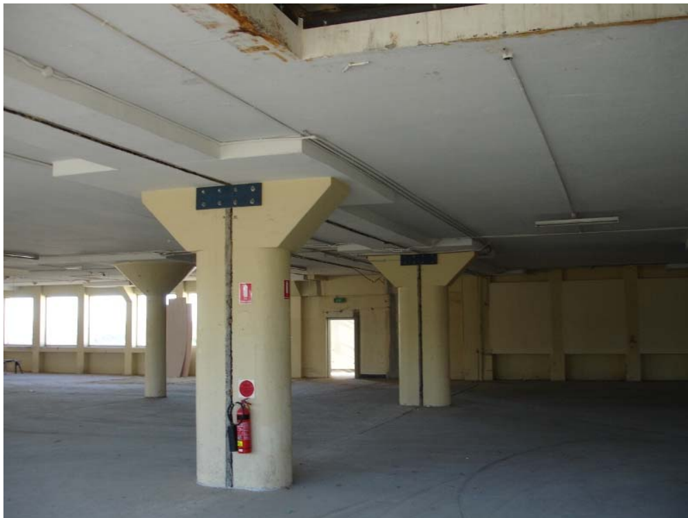
Photograph 24. Upper Ground Building Joint
