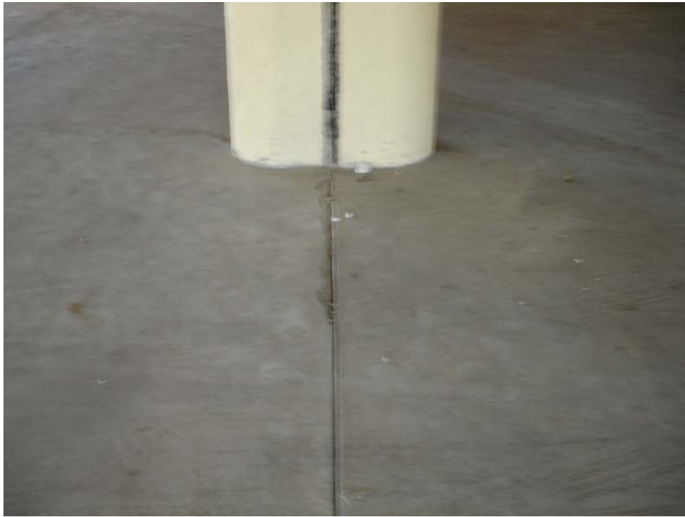
Photograph 29. Upper Ground Building Joint
