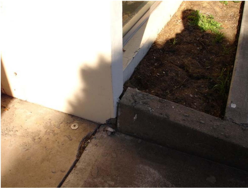
Photograph 15. Separation of concrete planter
