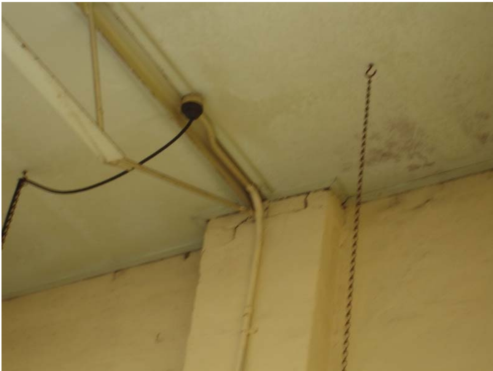
Photograph 48. Corrosion to truss bearing plate, cracking masonry
