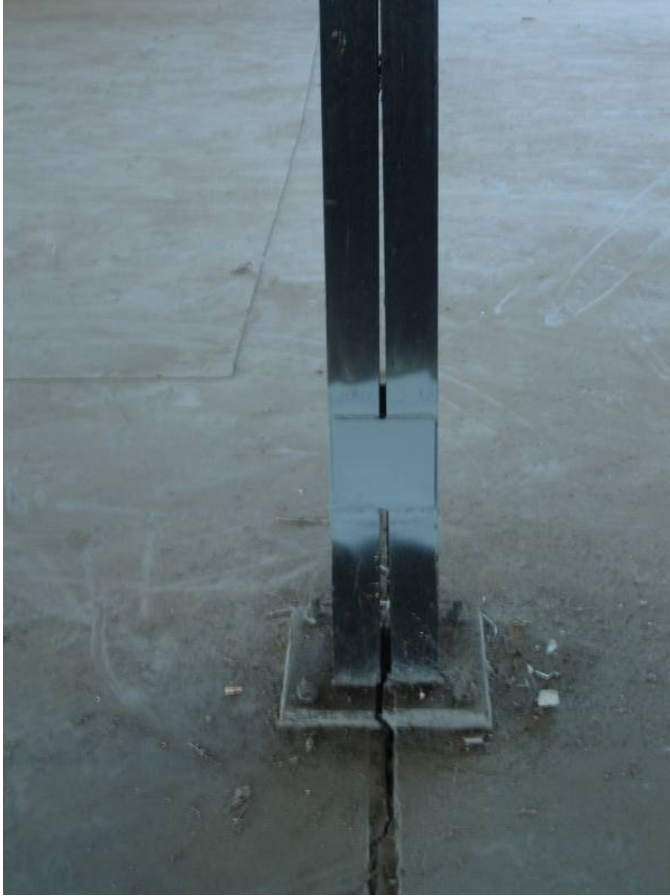
Photograph 45. Column built across building joint, previous repairs have occurred
