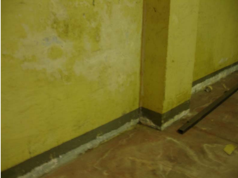
Photograph 32. Water Ingress Ground Floor, West Elevation
