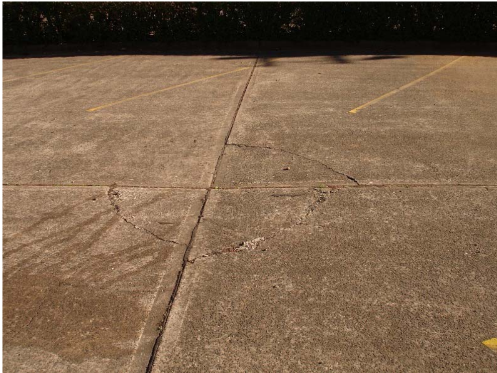
Photograph 17. Settlement and cracking of external pavement
