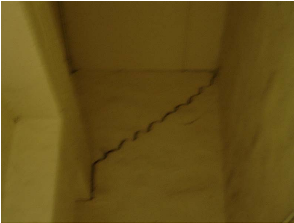
Photograph 47. Cracking masonry in stairwell
