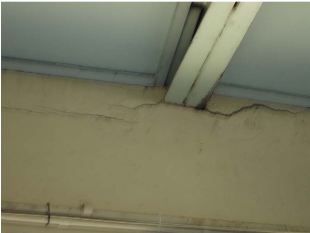
Photograph 44. Typical corrosion to truss bearing plate, cracking masonry
