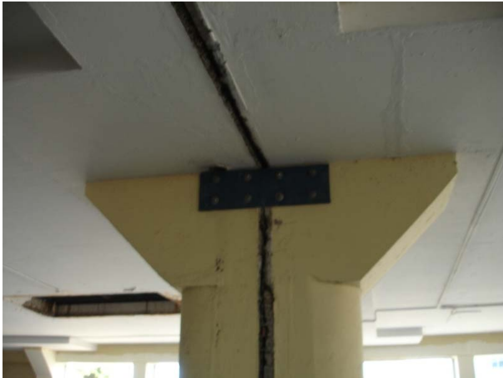
Photograph 27. Upper Ground Building Joint
