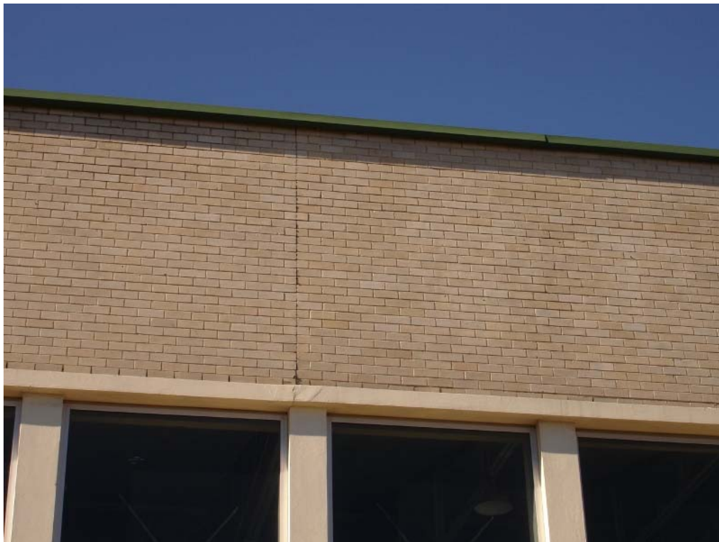
Photograph 18. Drummy render and cracking masonry at building joint, West Elevation
