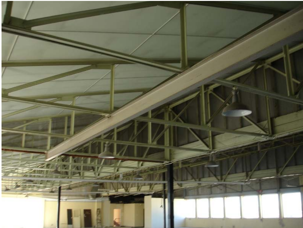
Photograph 41. Roof layout, no restraint to truss bottom chord
