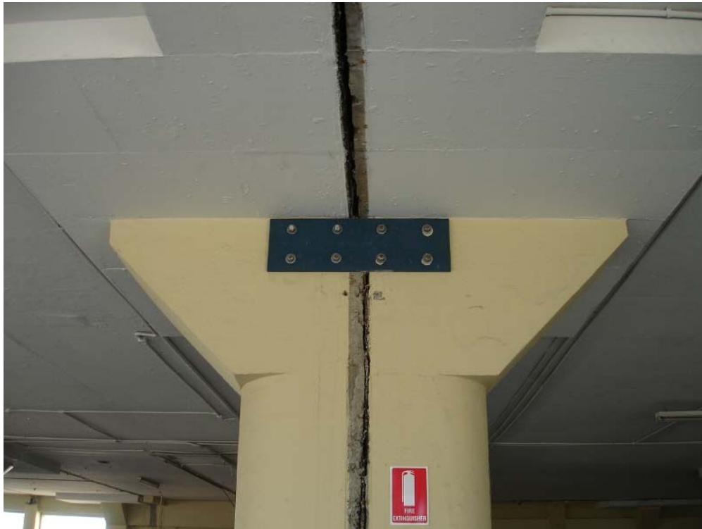
Photograph 25. Upper Ground Building Joint
