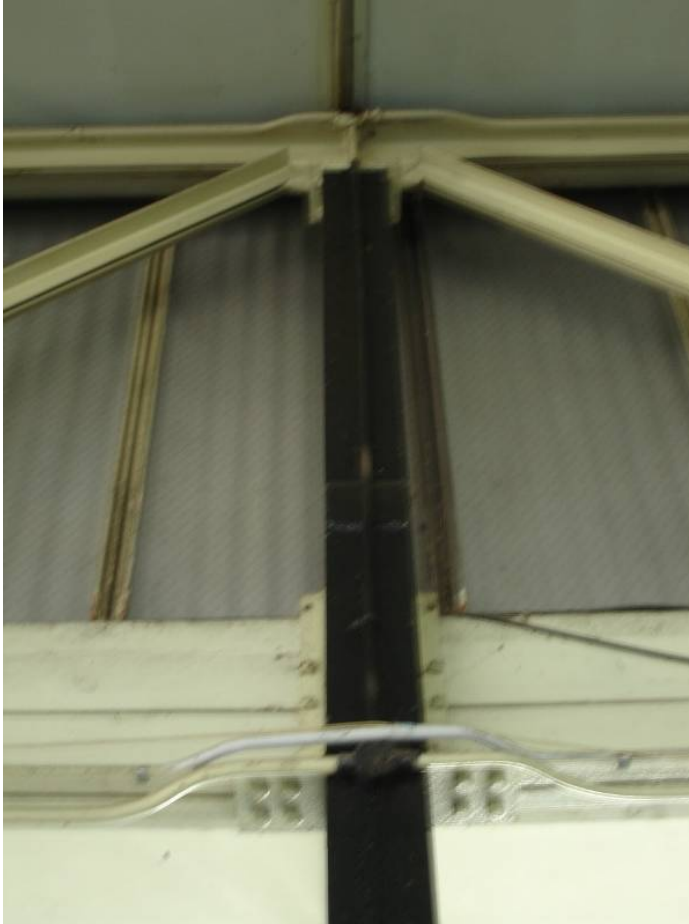
Photograph 46. Column built across building joint, previous repairs have occurred
