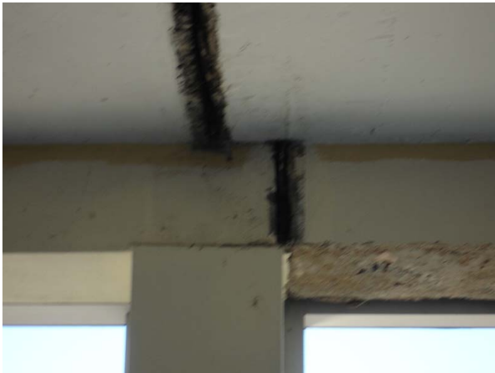
Photograph 26. Upper Ground Building Joint
