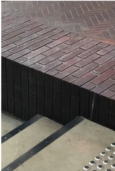
Brick wall - Kensington Street
