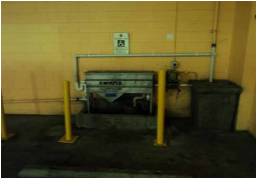
Photo 8 - Oil-water separator
