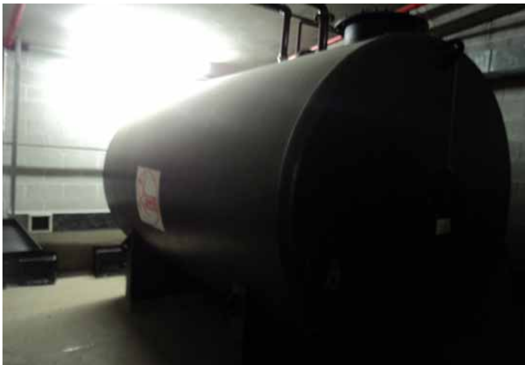
Photo 6 - Diesel tank underneath ramp
