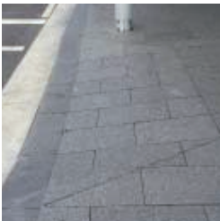
Kerb ramp Product: “Adelaide Black (Veined)” or “Austral Black” Size: 400x300x50, 200x300x50, 600x300x50mm Finish: exfoliated
