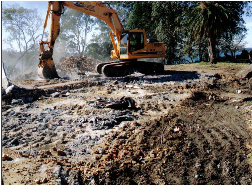
Plate 0.3 Machining removal of residual demolition debris and overburdens [Roll 1:9, facing E].
