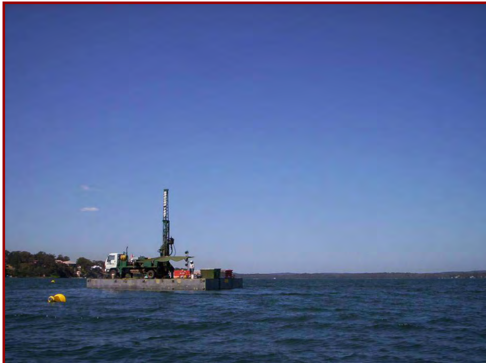
Photo 4 – drill rig set up on modular barge, in proposed marina area
