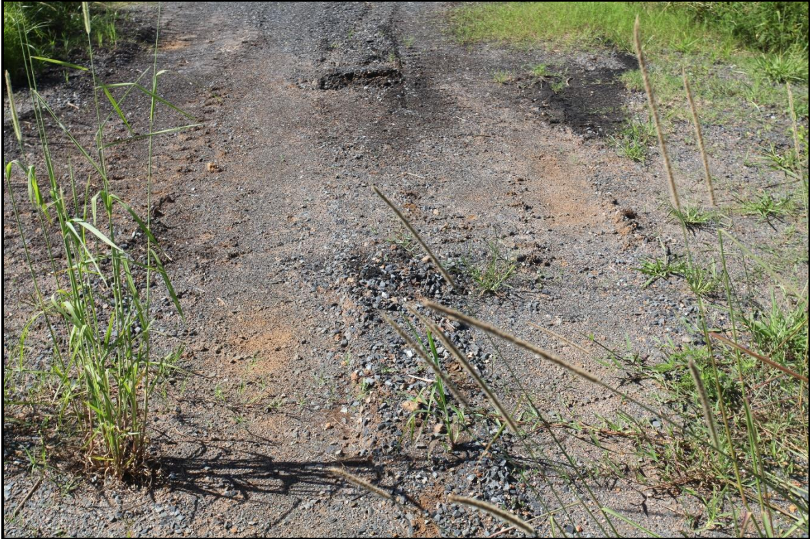
Figure 7: Remnant of fill and old gravel access.
