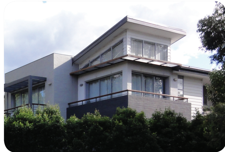
Window articulation to secondary street frontage
