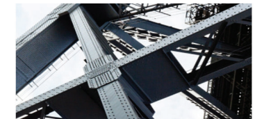
STEELWORK Steel to support balcony + roof
