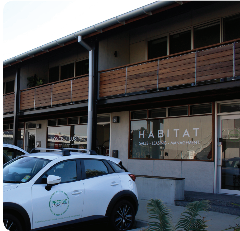
Building portico and separate entry path ensure the front door and work space are both legible
