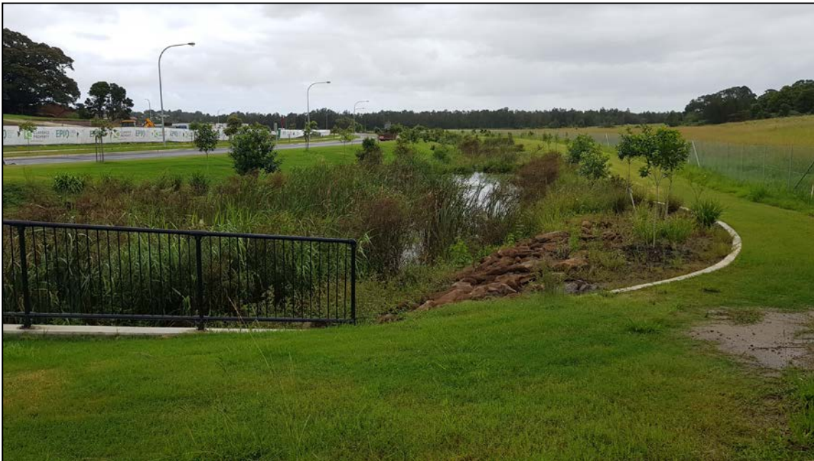
Plate 9. Typical view of re-engineered watercourse as constructed
