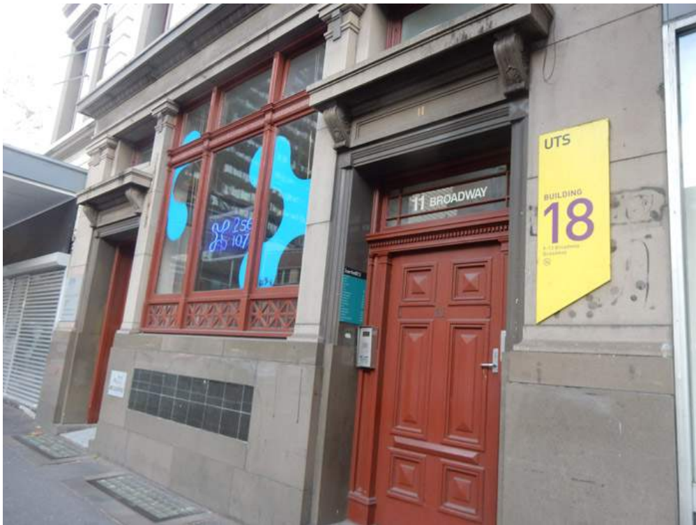
Figure 84: Shopfront to the former bank (formerly No. 11 Broadway), which is largely intact, note the pavement lights to the basement.
