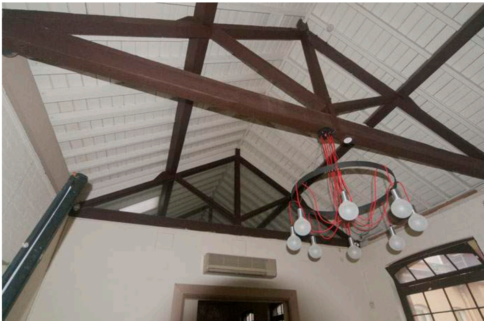
Figure 122: View of the 1 st floor level of former Apothecary building exposed roof framing and timber ceiling lining
