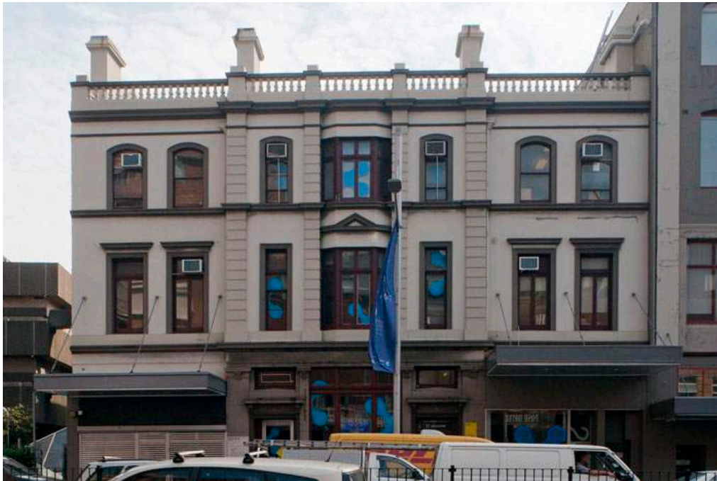
Figure 82: Front elevation in Broadway of the three retail terraces (from left to right, formerly Nos. 13 to 9 Broadway). Note modern awnings. Originally, the former Nos 9 and 13 had post-supported awnings, while the central former bank had no awning.
