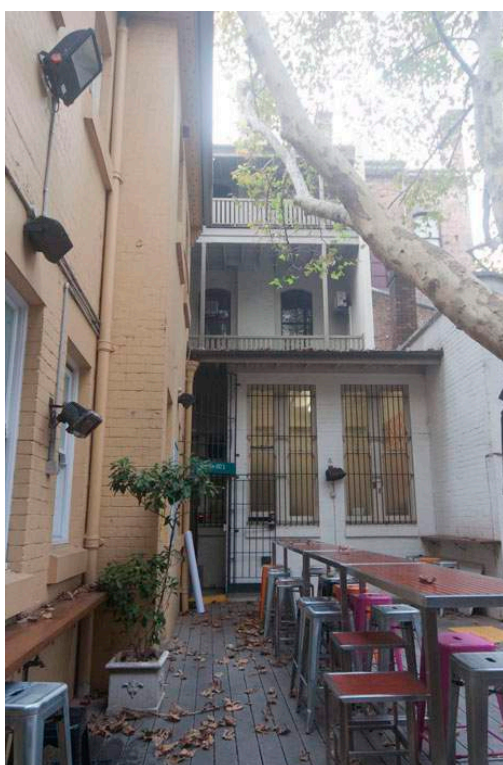
Figure 88: The rear wings of the former CBC bank (formerly No. 11 Broadway) and the rear wing of the former No. 13 Broadway. Note changes in the fenestration to the ground floor left and the alignment of a roof on the rear wall to the right.
