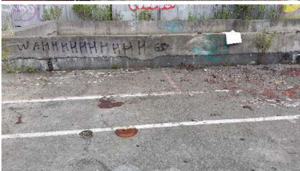
Photograph 12: South section of the site - Possible UST at the tank/bund.
