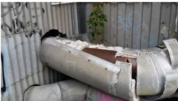
Photograph 8: P South section of the site – possible asbestos insulation at kiln / Furnace.
