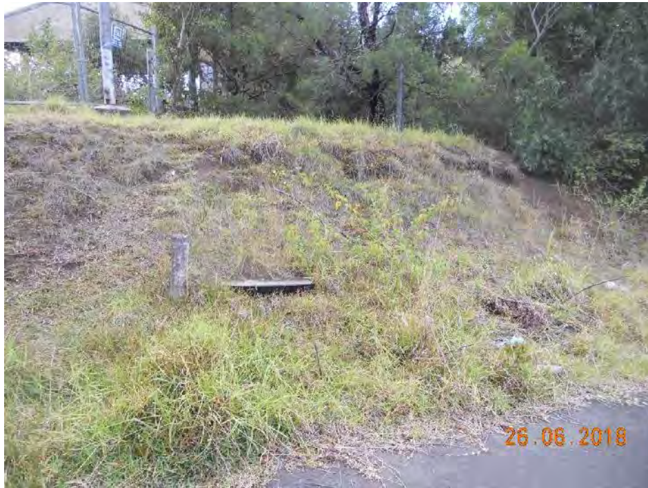
Photo 23 – 1.5 – 2m high cut batter exposing residual soils.
