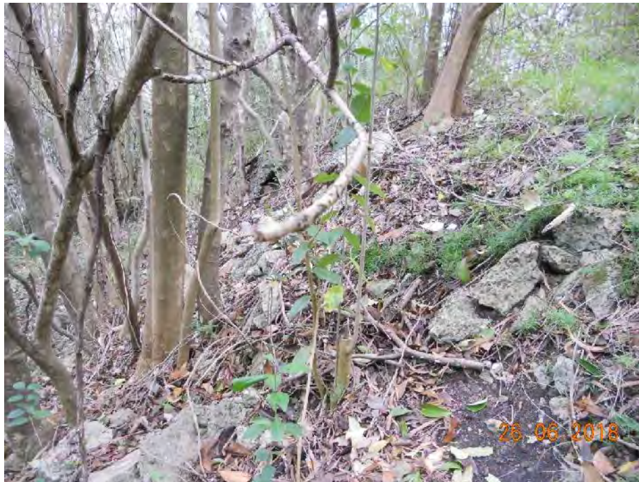
Photo 26 – Concrete pieces surface of batter probably formed with uncontrolled filling.
