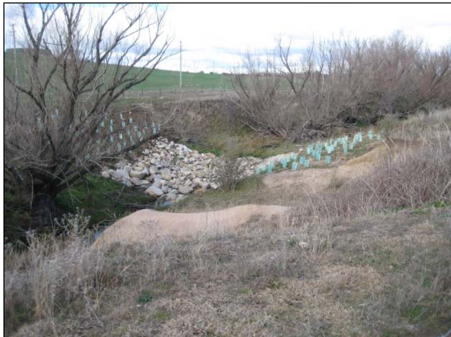
Photo 6: Rehabilitation works upstream of the site to prevent further head cuts.
