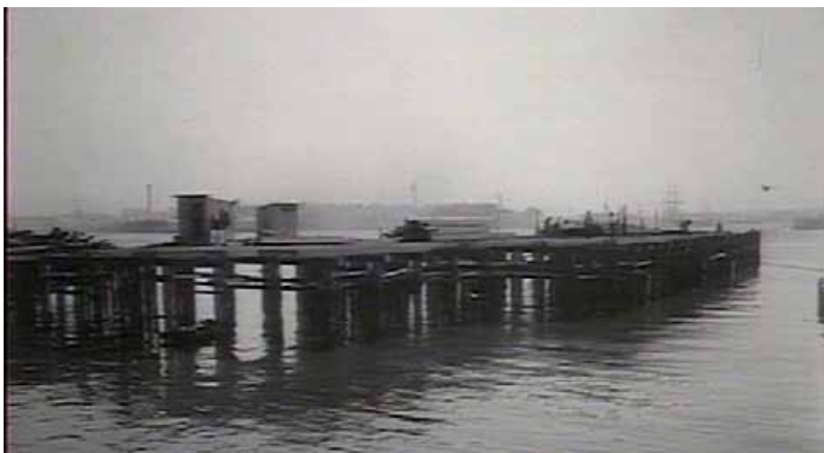
Figure 39. Construction of the Wharves on Turpentine Piles 78
