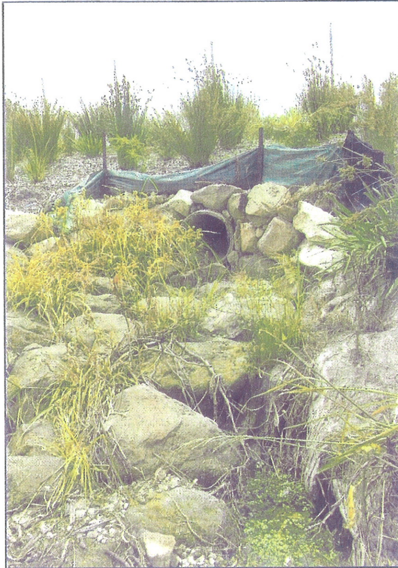
A riprap outlet on a steep slope. Source: SOILS AND CONSTRUCTION, Volume 1, 4 th Edition, March 2004, Managing Urban Stormwater, by LANDCOM.
