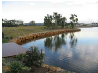
Various edge treatments to water detention ponds
