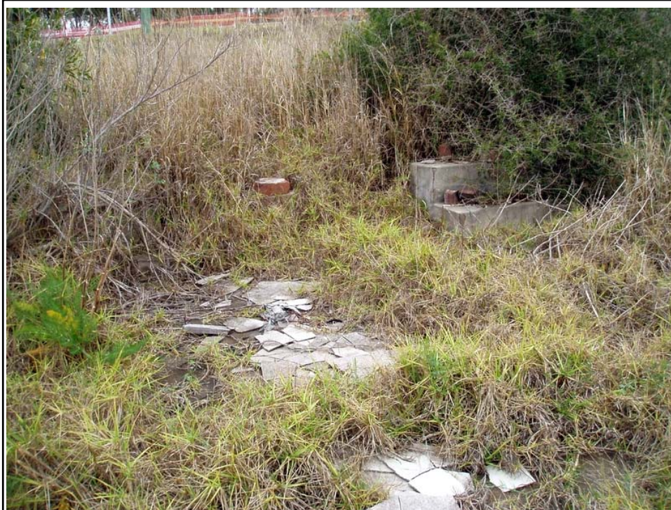
PHOTO 21: Remnant slabs and asbestos sheeting, from building demolition, Parcel 2.
