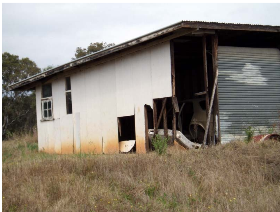
PHOTO 30: Fibre board structure (possible asbestos). Parcel 4.
