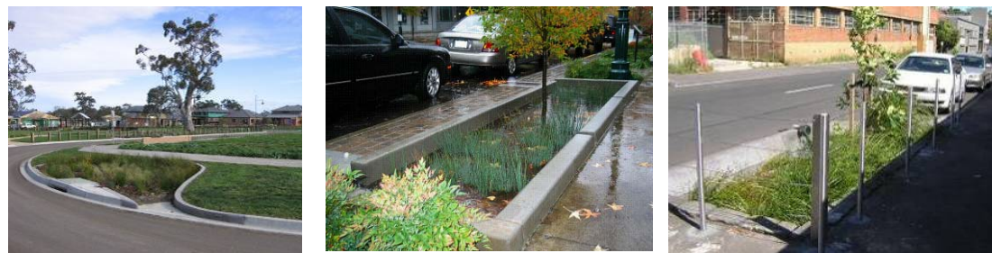
Figure 5-6 Examples of bioretention raingardens with streetscapes (parking bay type systems).
