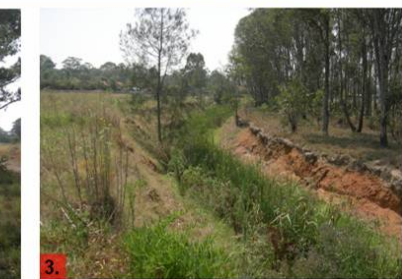
Constructed channel, redirecting stormwater from the culvert at Doonside Road to downstream section of the Northern Waterway (length 200m).
