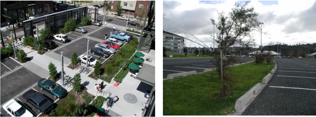
Figure 7-3 Green Car Parks – with shading, bioretention systems and careful material selection
