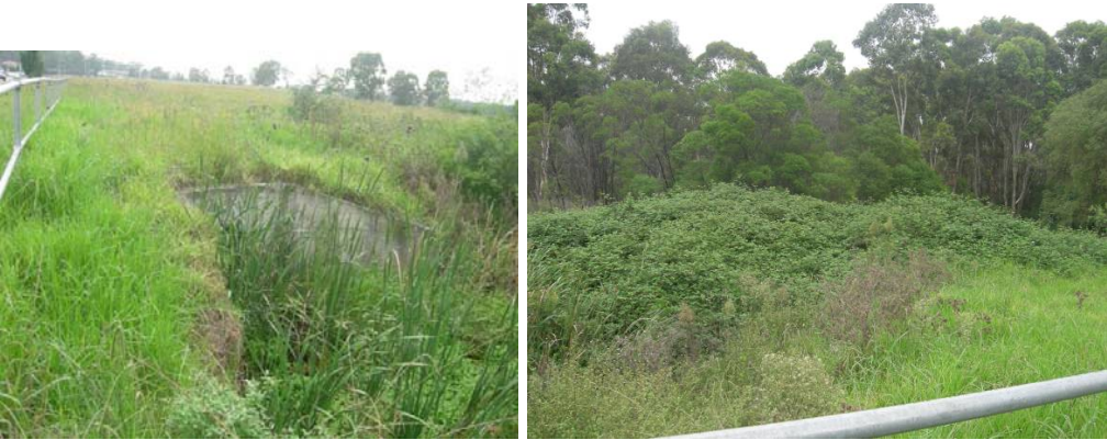
Figure 2–4 Weed growth and disturbance due to uncontrolled discharge of stormwater
