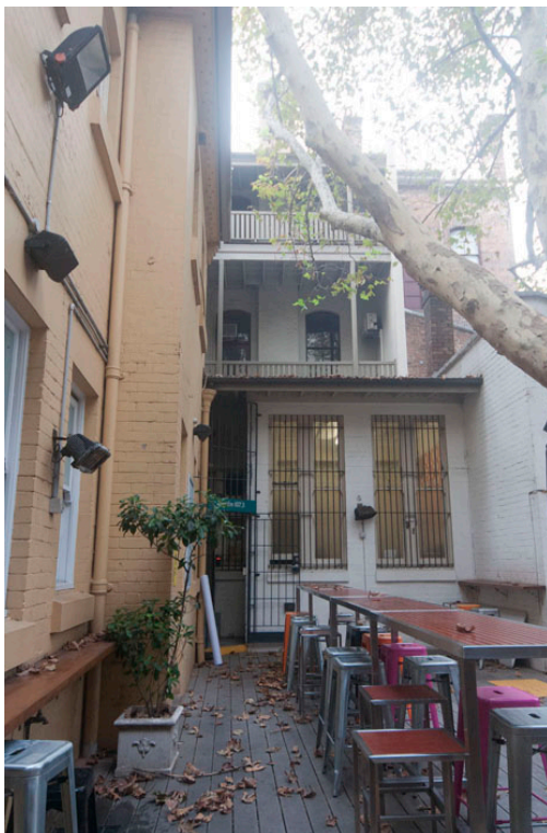
Figure 92: The rear wings of the former CBC bank (formerly No. 11 Broadway) and the rear wing of the former No. 13 Broadway. Note changes in the fenestration to the ground floor left and the alignment of a roof on the rear wall to the right.
