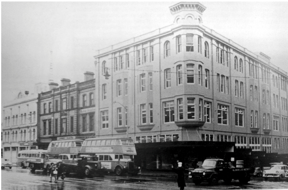
Figure 43: The former store in 1965 and after alterations for conversion into uses by the Sydney Technical College. Associated with this conversion probably was the cement rendering of the facades, and changes to the detail of the parapet. The timber framed sashed windows appear to date from the 1909 build. Source: Neill, N, Technically & further: Sydney Technical College, 1891-1991 , Hale & Iremonger, 1991, p.100
