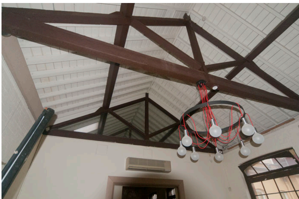
Figure 126: View of the 1 st floor level of former Apothecary building exposed roof framing and timber ceiling lining
