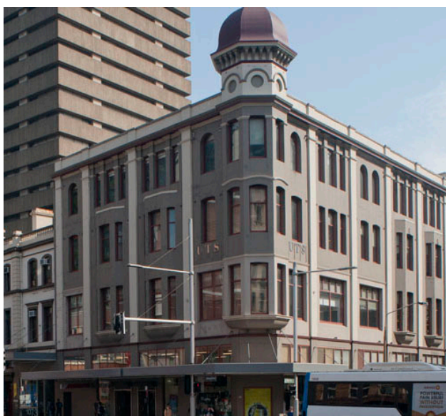
Figure 56: The Bon Marche store today. Note loss of original awning & shopfronts, cement rendering of walls, removal of parapet decorative detail. Though not visible in this photograph, the cupola still retains its apex flagpole. The current colour scheme changes the visual presentation of the building from the original brickwork by adding emphasis to the vertical pilasters and parapet.
