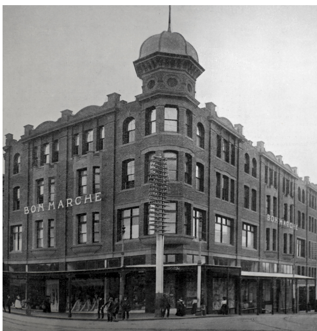
Figure 55: The Bon Marche store as completed in 1909. Source: The Salon , March 1914. Note the face brickwork and window head and sill detailing and the posted street verandah. The brickwork is monochrome and not patterned. The built form is restrained and has very little ornamentation or decoration.
