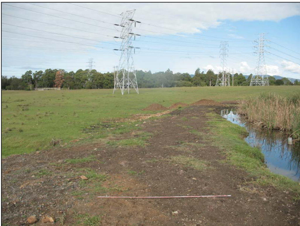
Plate 2 Disturbance associated with the construction of dams, facing west
