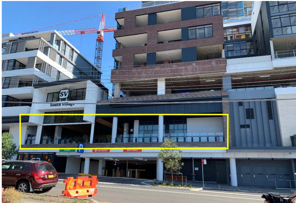
Figure 2 – Photograph of South Village Shopping Centre: Southern elevation to Flora Street to be altered
