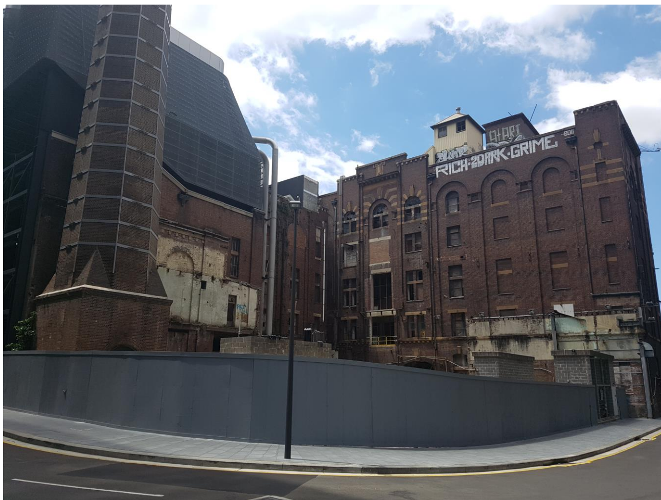
Figure 5 Existing Brewery Yard building and site conditions
