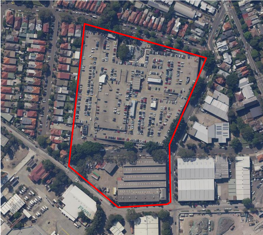
Figure 1 – Aerial view of the site (outlined in red)
