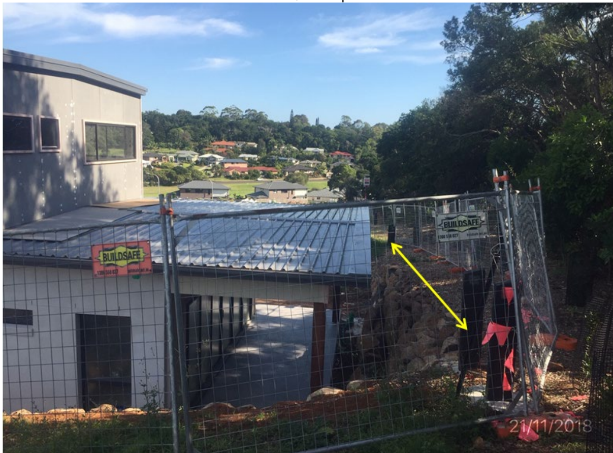
Plate 3: Existing conflict between new residential dwellings and retained rainforest (Zone 2) within the EPIQ development. Landholder has now requested removal of some of the existing rainforest. Problems will increase as newly planted vegetation matures. Yellow line depicts edge of restoration area.
