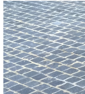
Granite Setts - loading bay
