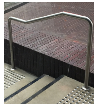
Steel handrails + TGSI. AS1428.1 compliant
