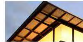
EAVES DETAIL Exposed hard wood timber framing; Galvanised Trimdek roof sheeting
