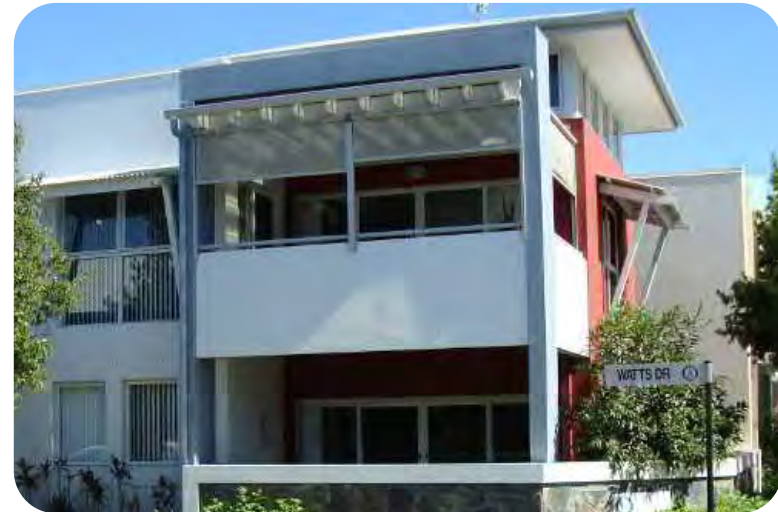
Balconies encouraged on secondary street frontages
