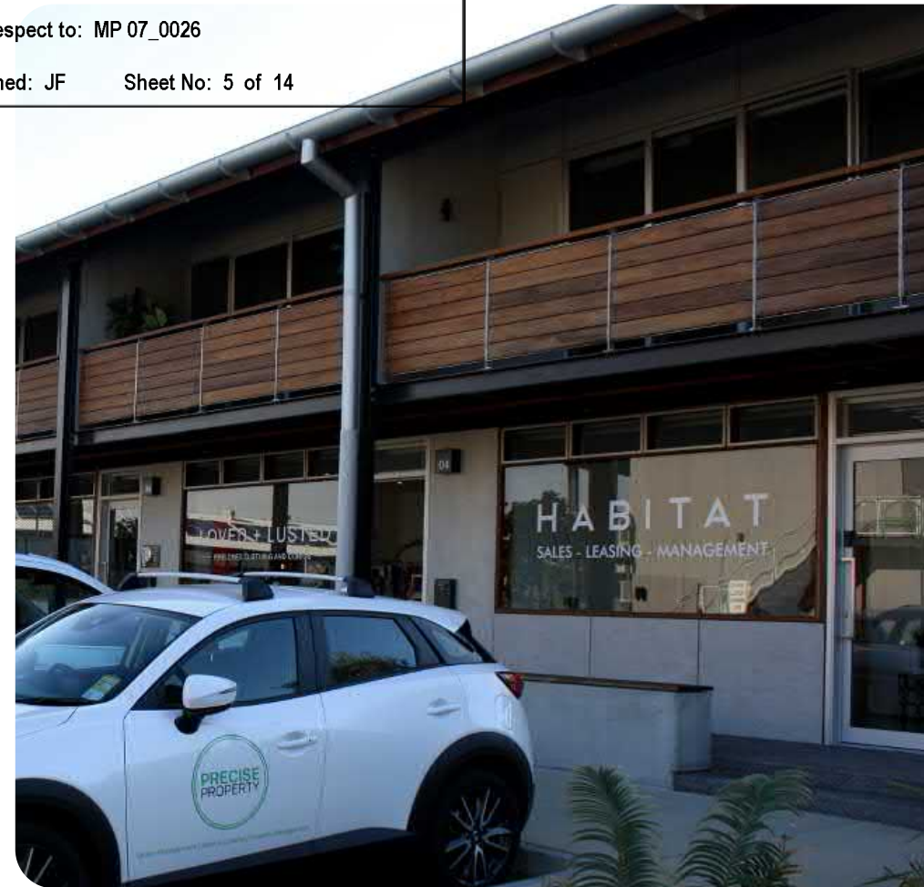
Building portico and separate entry path to ensure the front door and live/work spaces are both legible
