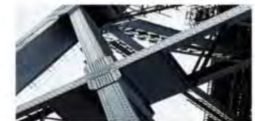
STEELWORK Steel to support balcony + roof
