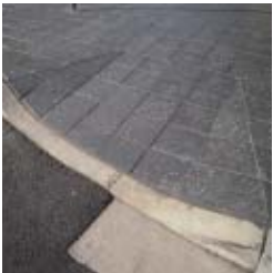
Kerb ramp Supplier: Pebblecrete Product: PPX:544:35D Size: 300x300x60mm Finish: shotblast
