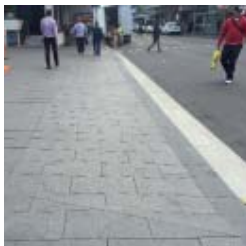
Vehicle crossing Product: “Adelaide Black (Veined)” or “Austral Black” Size: 400x300x50, 200x300x50mm Finish: exfoliated
