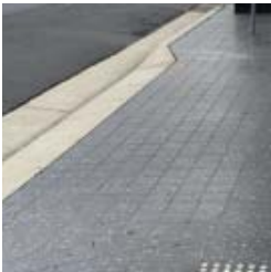
Vehicle crossing Supplier: Pebblecrete Product: PPX:544:35D Size: 150x150x60mm Finish: honed
