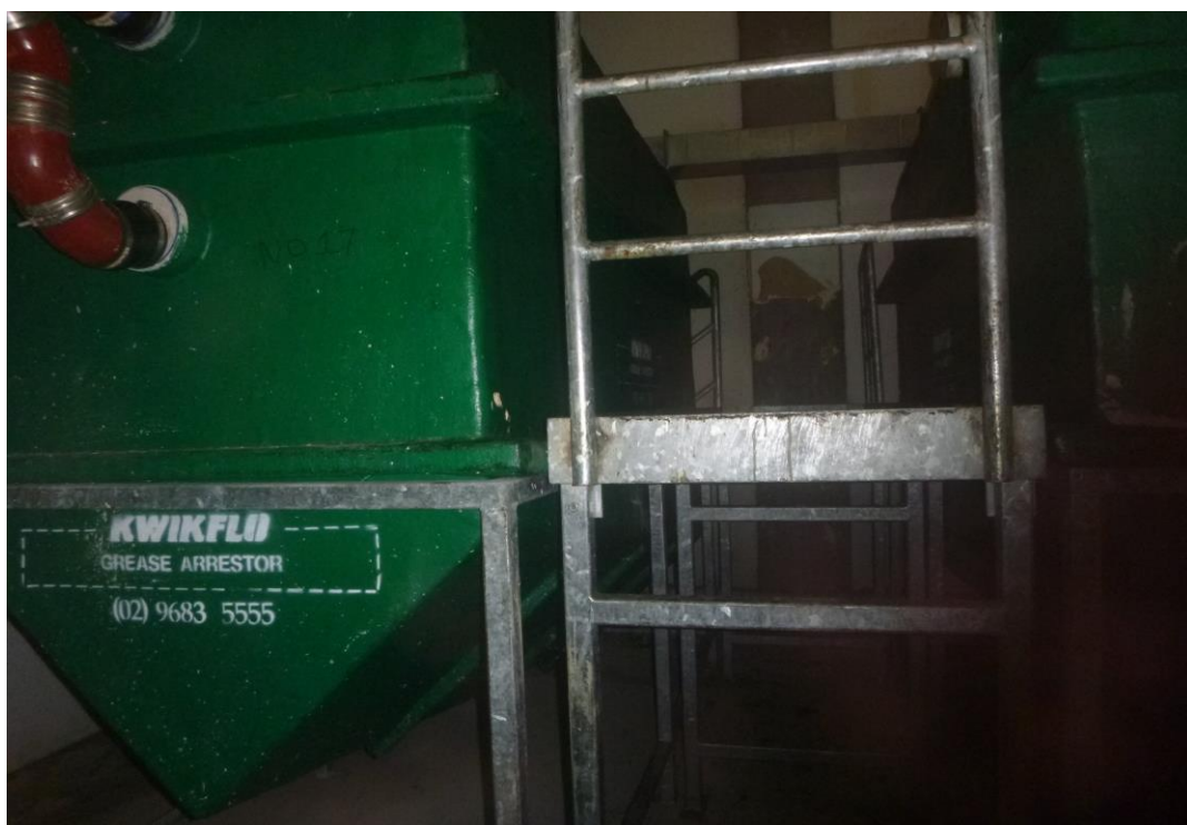
Photograph 5 - Above ground grease traps
