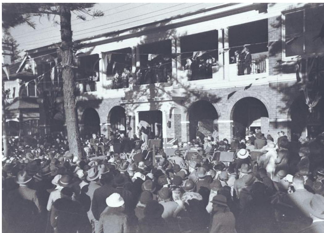
Source: State Library of NSW, Image No. Home and Away – 4924 by Sam Hood
