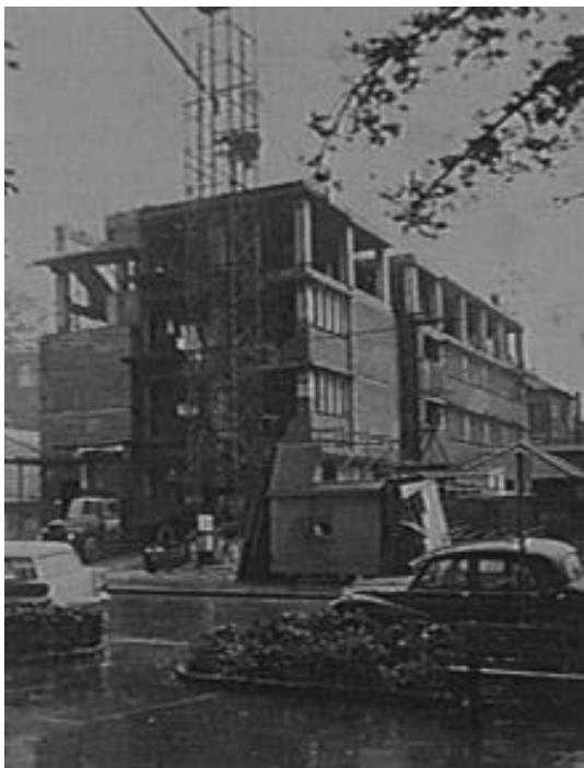
Figure 19 – Construction of the Moncrieff Barron Wing, 1964
