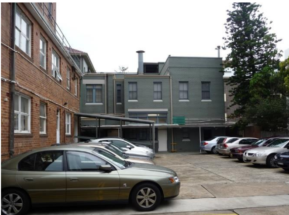
Western elevation of rear 1960s addition to Drummond House and Elsie Hill building (left) with rear car park
