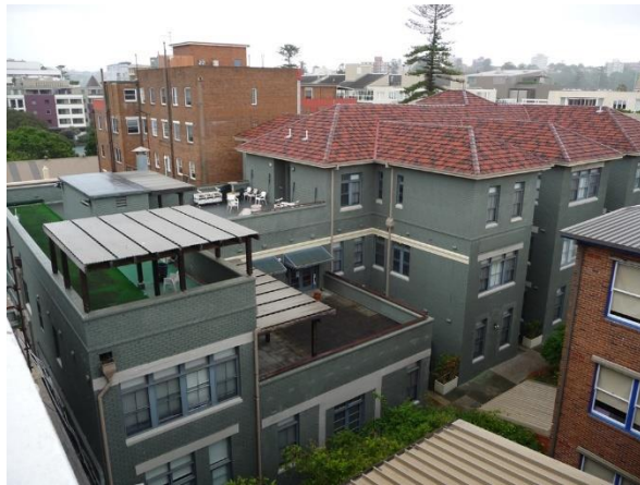
Roof and rear extension
