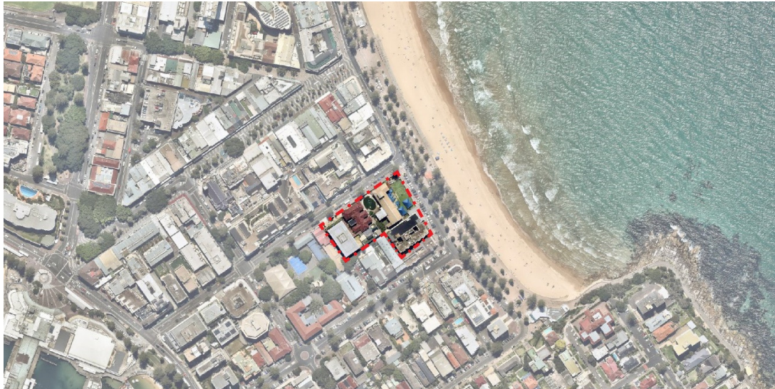
Figure 1: The subject site. Source SIX Maps NSW; https://maps.six.nsw.gov.au
