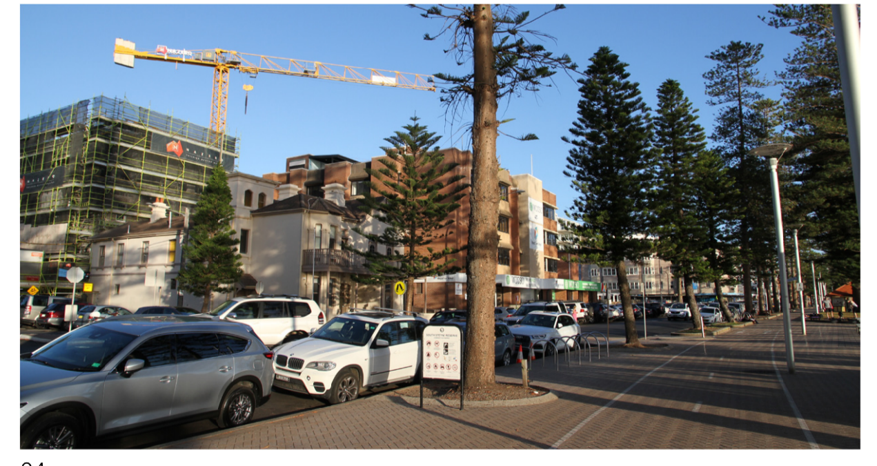
04. PART VIEW OF SUBJECT SITE FROM SOUTH STEYNE LOOKING NORTH WEST.
