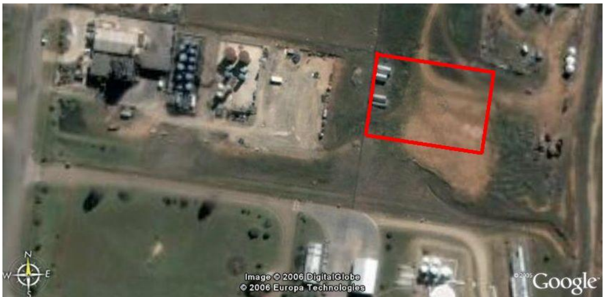
Figure 2: Aerial photograph of the site, with new tank farm area indicated in red
