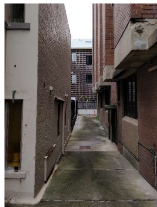
Figure 26: Photography looking toward the subject window (level 1) at No 29 Victoria Pde.
