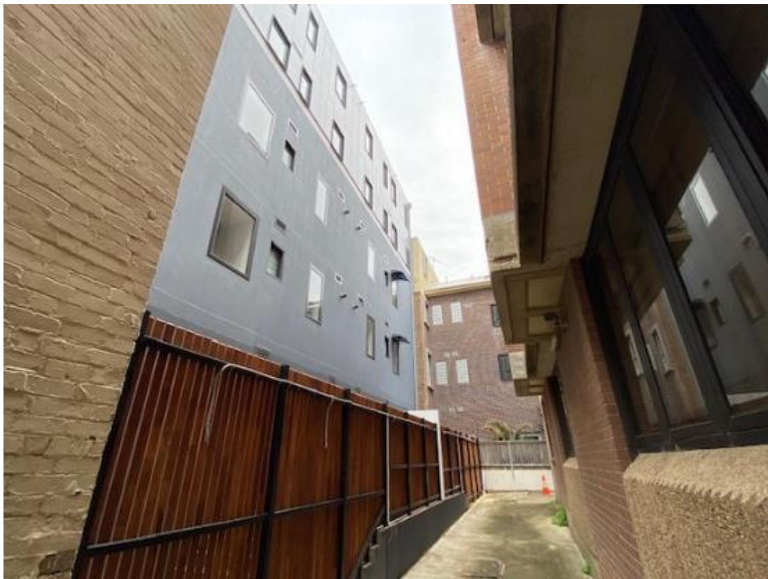
Figure 3 - View looking west down southern boundary between No. 31 Victoria Parade and proposed Building C
