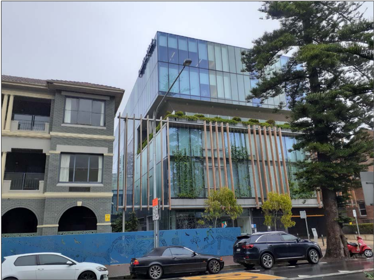
Figure 3 | Recently constructed CCK building adjacent to Drummond House (Source: Department's photograph)
