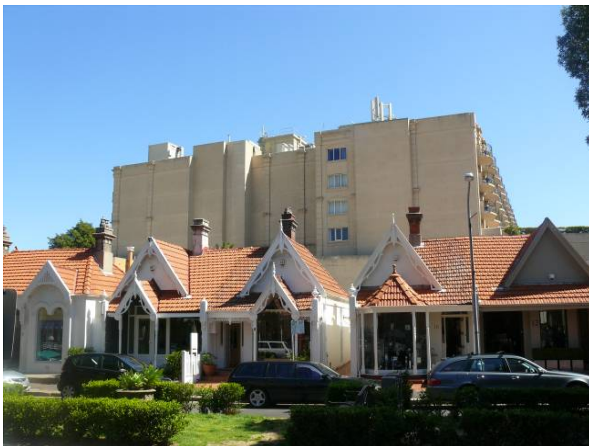
Figure 59. Site as viewed from Transvaal Avenue
