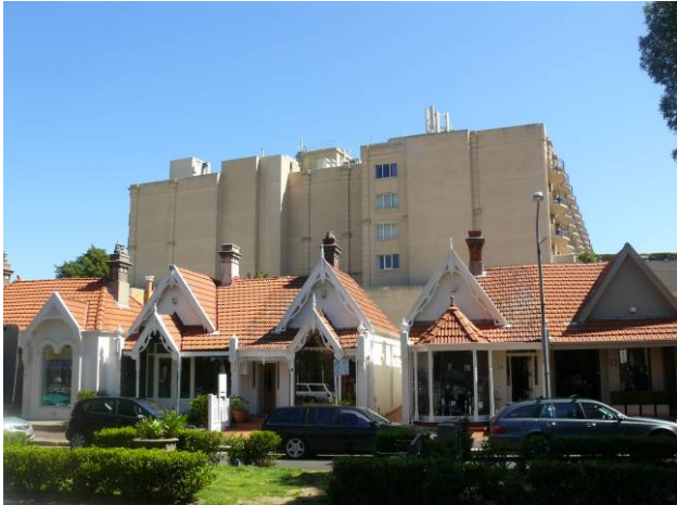
Figure 15. View from Transvaal Avenue to the east The building presents as a 6 storey (equivalent of 7-8) residential stories to the east. This monolithic form presents as a bulky and massive backdrop to the Conservation Area.
