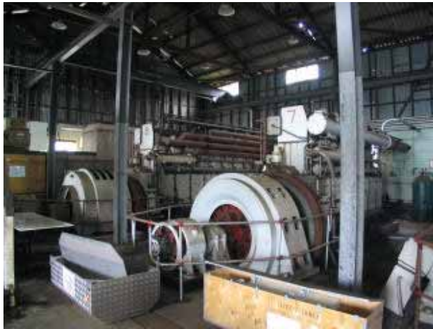
Photograph 3.6 The Mirrlees units 7 and 8 located east of the No. 6 unit. Mirrlees unit 8 is fitted with the Schorch alternator
