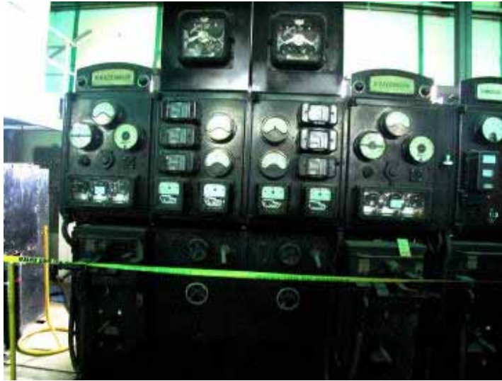
Photograph 3.33 Control panel for the No.8 and No. 7 alternators
