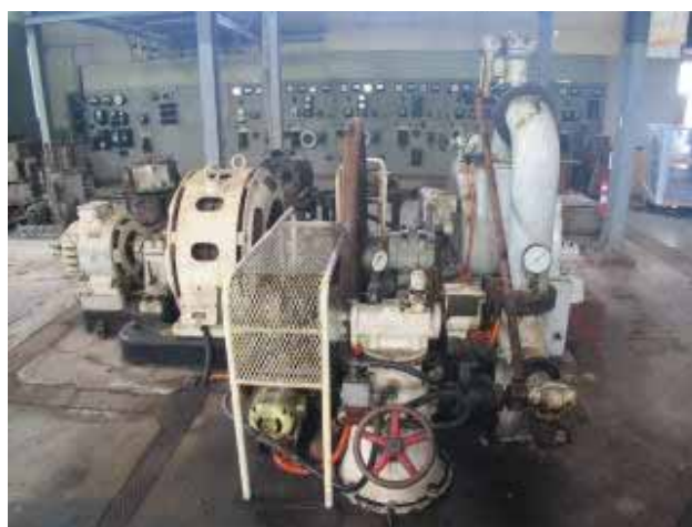
Photograph 3.2 The No.s 1 and 2 hydro units with the control panel behind
