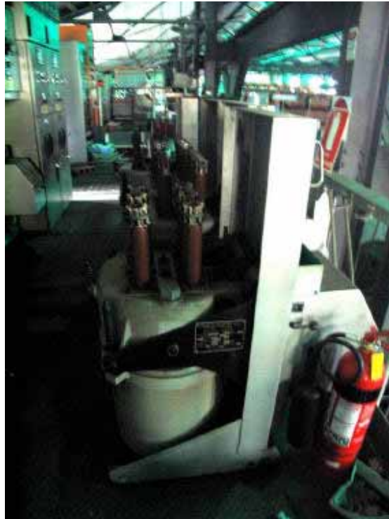
Photograph 3.31 English Electric Oil Circuit Breakers on the mezzanine
