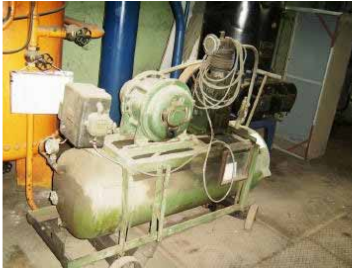
Photograph 3.27 Australian General Electric induction motor located adjacent to Unit 6
