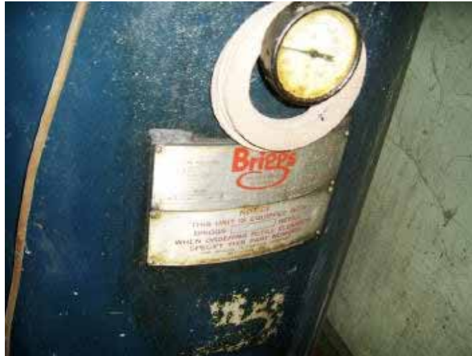
Photograph 3.23 The Briggs starting air receiver for Unit 8
