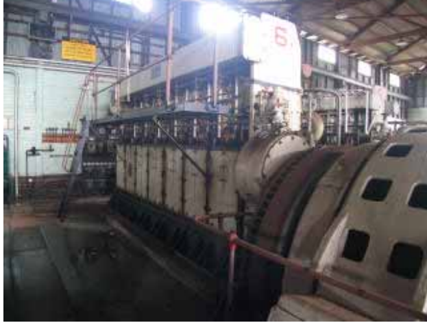
Photograph 3.5 The No. 6 Mirrlees engine (Note water pooling on the floor)
