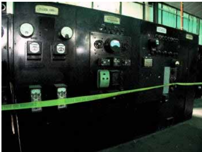
Photograph 3.34 Metering panel and voltage regulator
