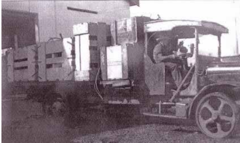
Figure 2.5 Delivery of machinery to the Lismore Power Station c1932 – the photograph is annotated with the caption: This is one of the first consignments of machinery being delivered to the new power house consisting of two of the Engine Cylinders each weighing 3 tons each, P Oakes South Lismore
