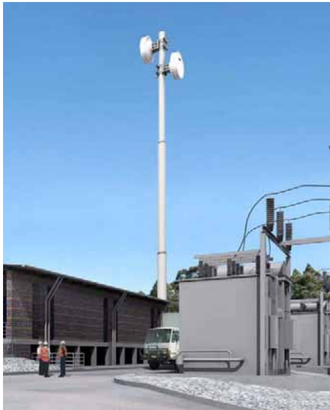
Figure 3.6 Example of slimline communications pole with dish antenna
