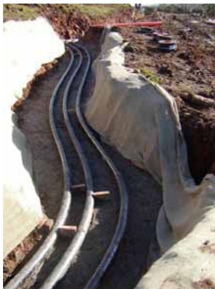
Figure 3.13 Indicative Photograph of the Installation of Underground Conduits
