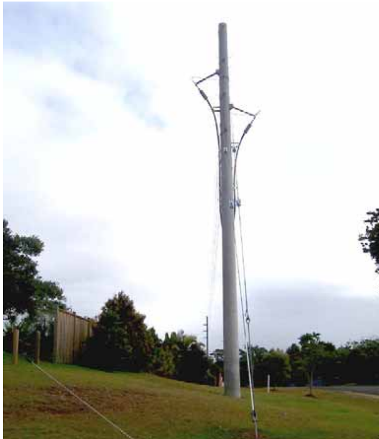
Figure 7.2 Example of Overhead to Underground Transition Infrastructure
