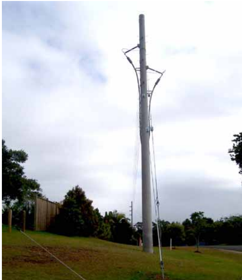
Figure 3.2 Example of Overhead to Underground Transition Infrastructure
