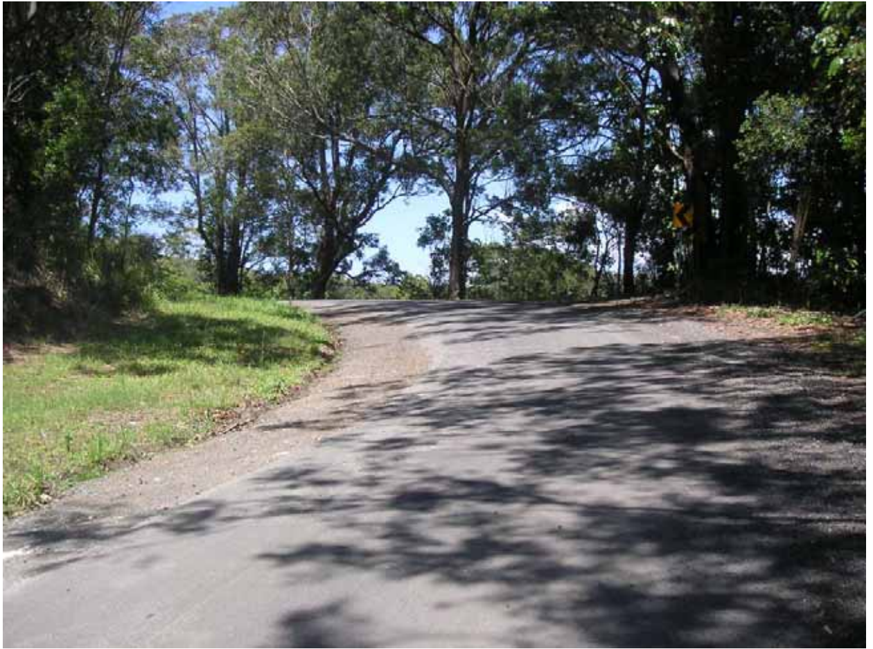
Photo 4: View of Skinners Shoot Road looking toward the south from approximately CH 231 showing the start of the first of the realignment works that will be required between CH 231 – 317 involving adjustment of the pavement cross fall and horizontal road alignment. This is the steepest part of the proposed access drive being in the vicinity of 10 degrees.
