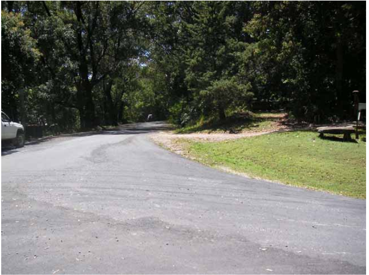
Photo 9: View of Skinners Shoot Road where it intersects with Yagers Lane, looking to the North of current access arrangements between CH 1508 (stn 29) – CH 1444 . The formation at this section will also require adjustment of the pavement cross fall and horizontal road alignment for low loader turning arrangements.
