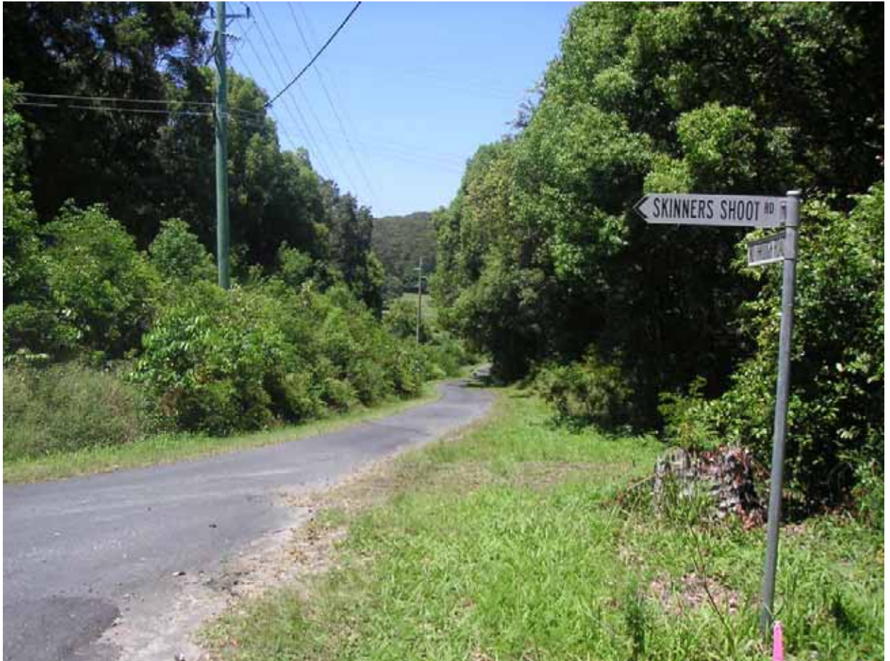
Photo 10: View of intersection of Skinners Shoot Road & Yagers Lane looking toward the east in the direction of the entrance to the Yagers farm site. This section of road will require environmental control, repair and extension of existing pipe culverts, excavation and widening of the road shoulders and overlay of existing pavement with 100mm road base. The two coat flush seal and minor reshaping will benefit the use of the Yager's farm as a nursery and reduce maintenance in the long term associated with the substation (and to protect against scouring in larger storm events).
