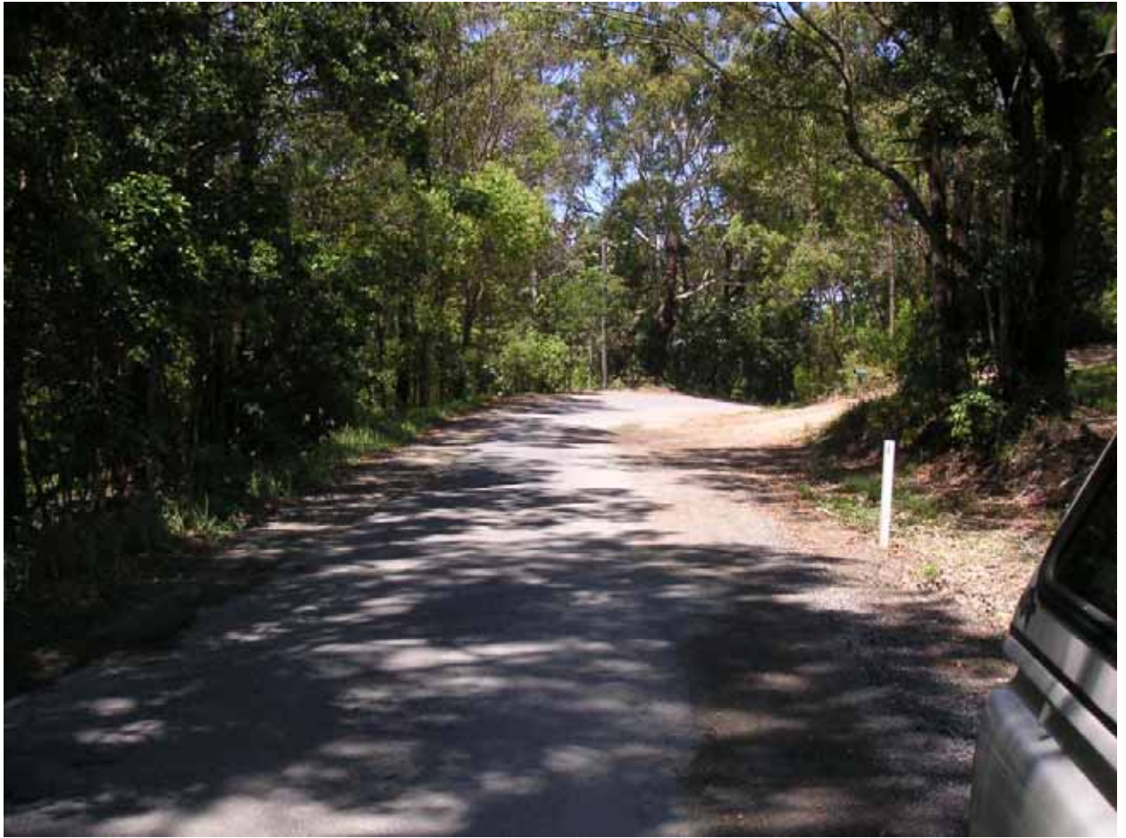
Photo 7: View of Skinners Shoot Road looking toward the south east from about CH 522 showing start of the next section of realignment works which will be required between CH 548 – 611 involving adjustment of the pavement cross fall and horizontal road alignment.
