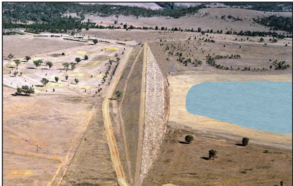
Subsidiary dam wall raising
